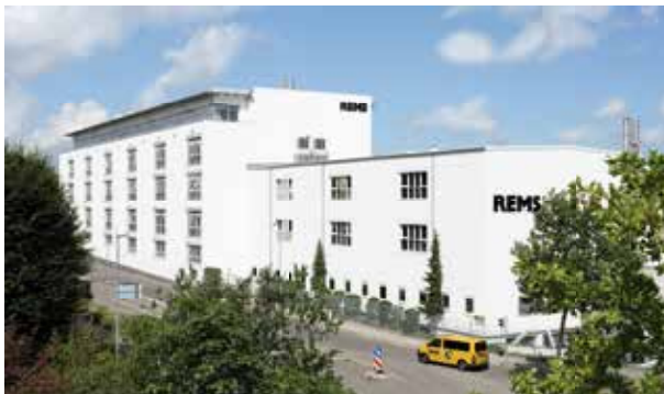
REMS training centre in Waiblingen near Stuttgart.
